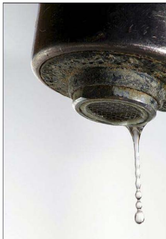
Limescale buildup from hard water can be seen on the faucet shown in the photo above.
